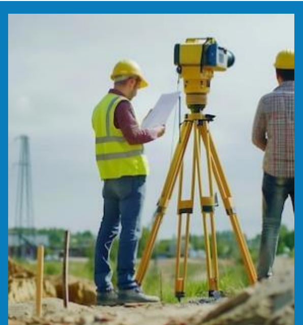
Survey and Soil Investigation
