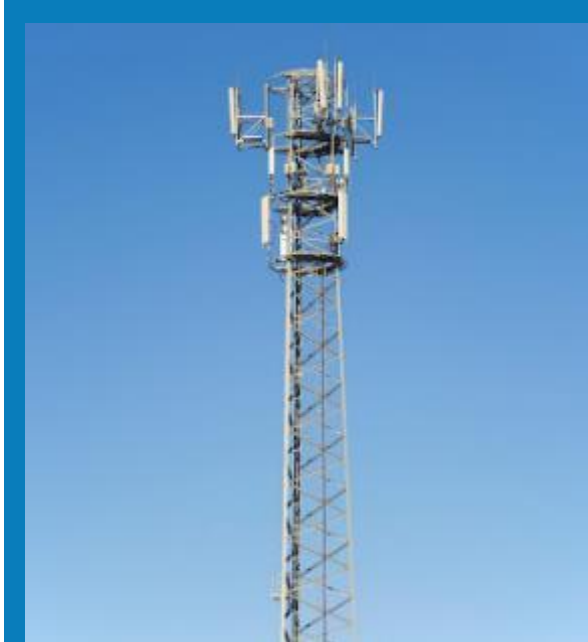
Telecommunication Towers Erections
